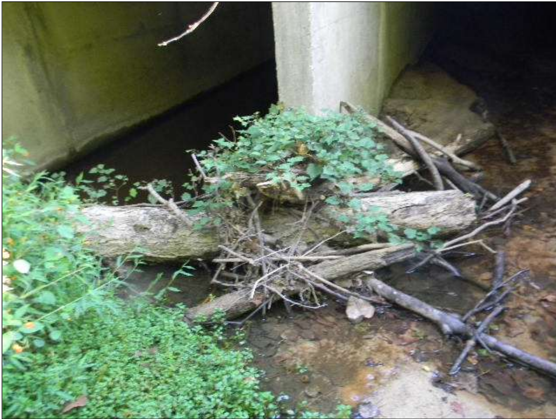
15' WIDE X 3' HIGH X 4' DEEP DRIFT ACROSS THE INLET OF BARRELS 1 & 2.
