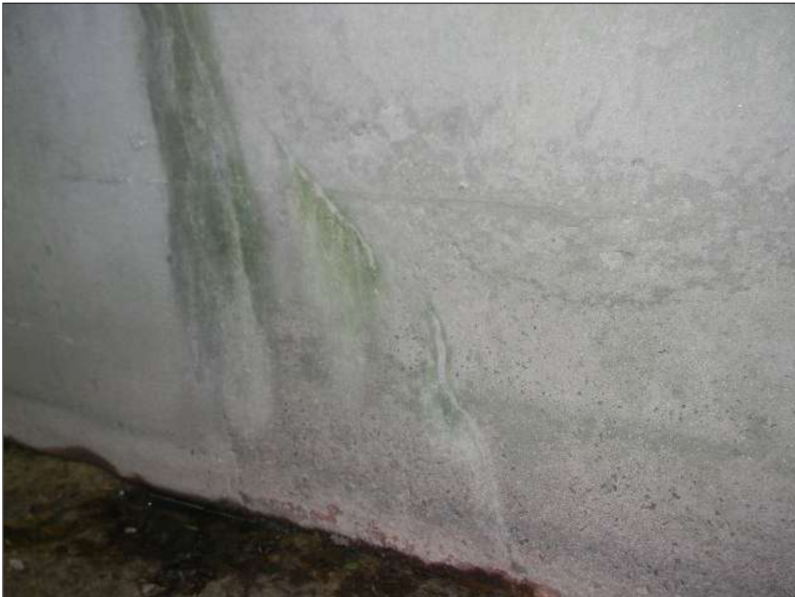
EXTERIOR WALL 2 HAS A 6' LONG DIAGONAL CRACK NEAR THE OUTLET EXTENDING FROM THE CONSTRUCTION JOINT.
