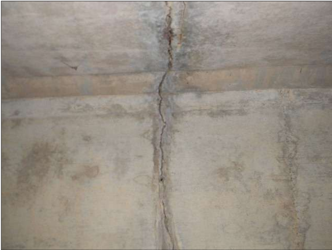
CONSTRUCTION JOINT AT 70' FROM THE INLET IS CRACKED AND OPEN 1/4" IN THE TOP SLAB AND WALLS.
