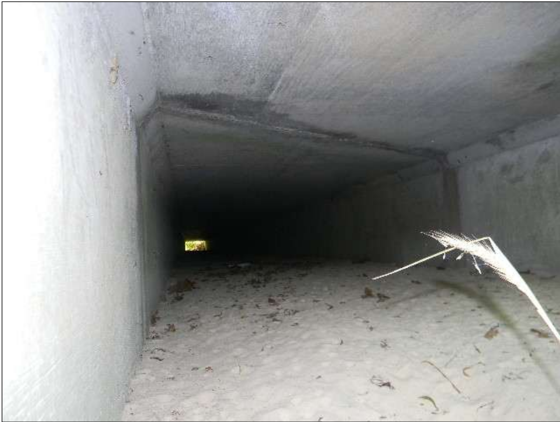
6' SEDIMENT BUILDUP IN BARREL 1. BARRELS 2 & 3 HAVE 2' SEDIMENT.
