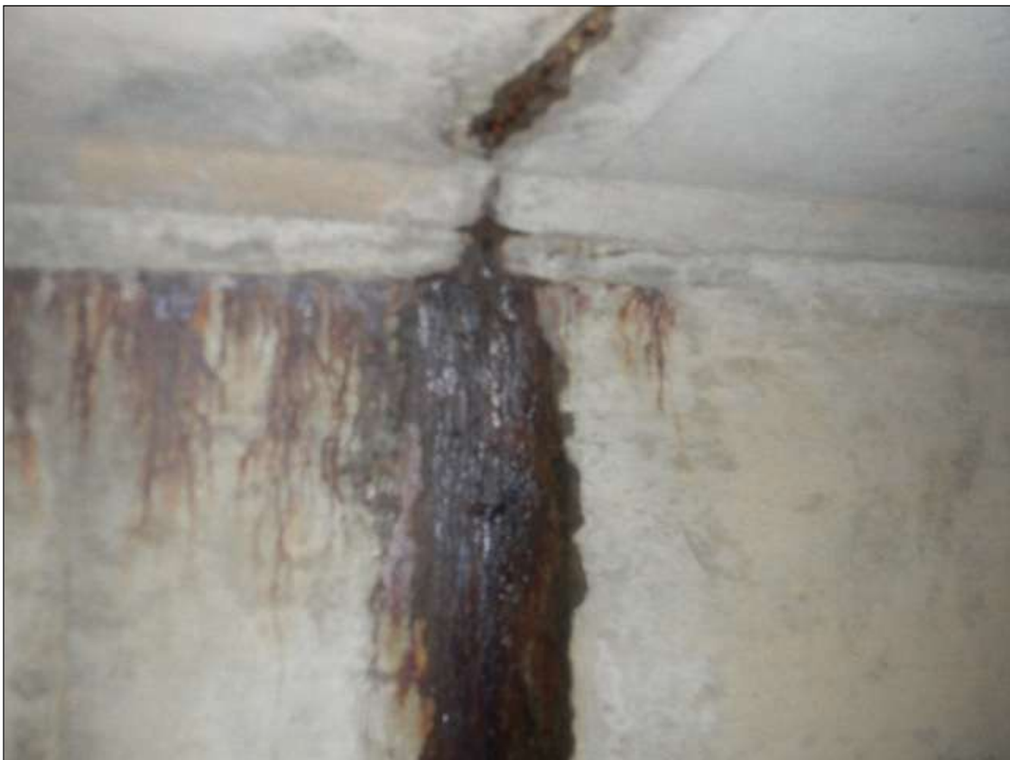
CONSTRUCTION JOINT AT MIDSTRUCTURE IS CRACKED AND LEAKING.
